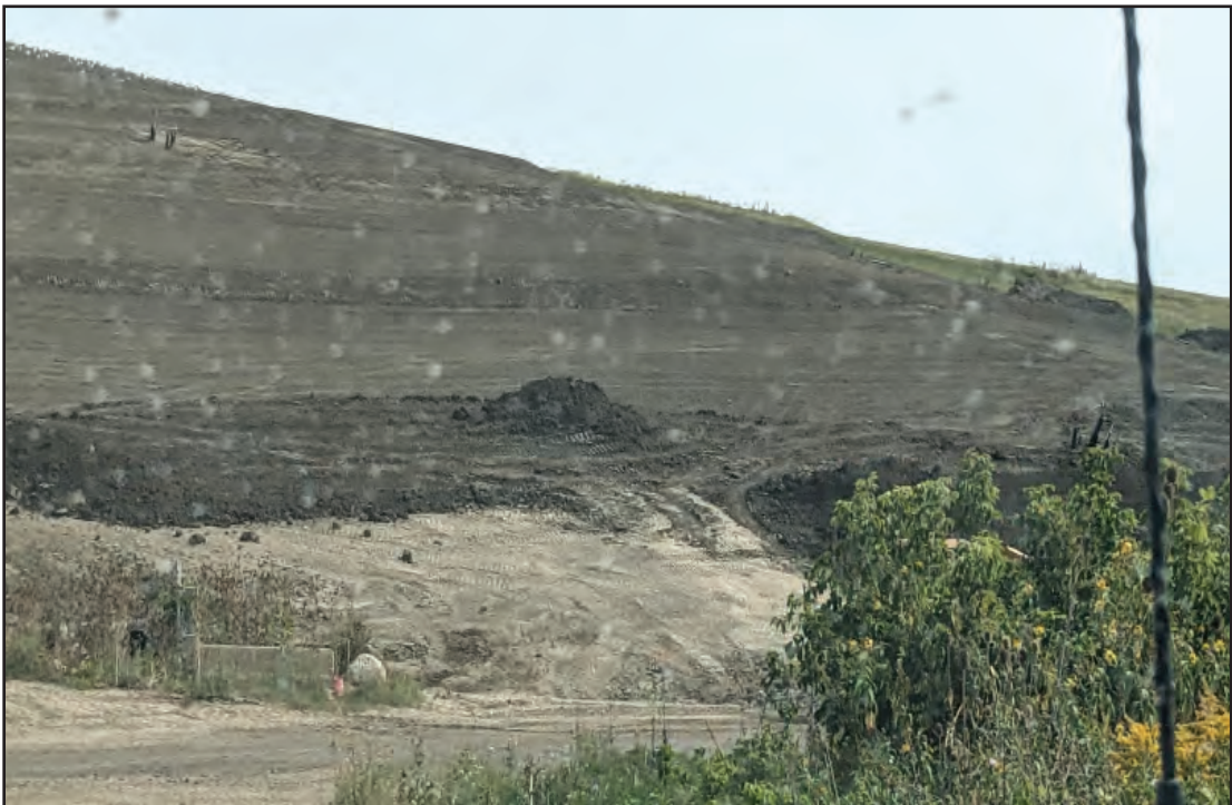
Top soil placement on new cap nearly complete
