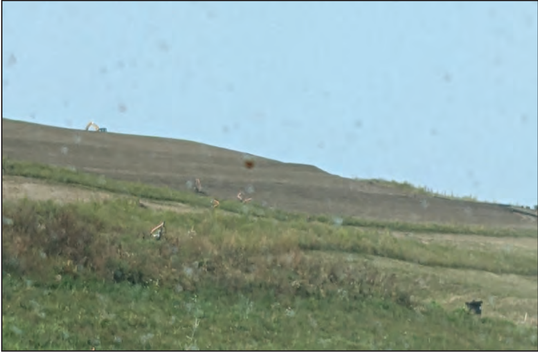
Cap cover soils over plastic cover
