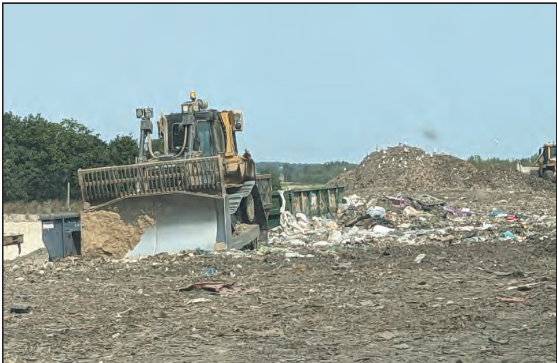
Travelway in active area improved with wood waste
