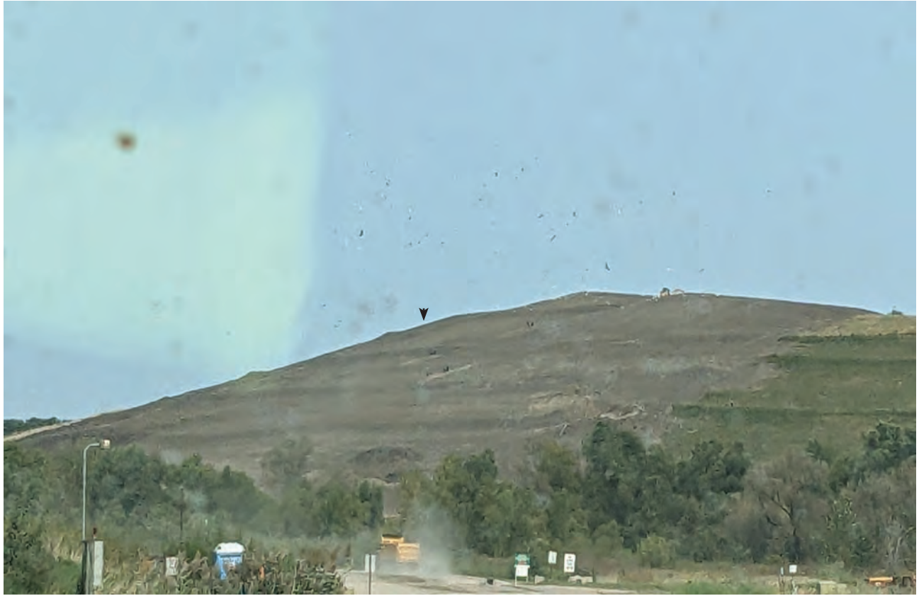
New cap nearly complete with top soil placement
