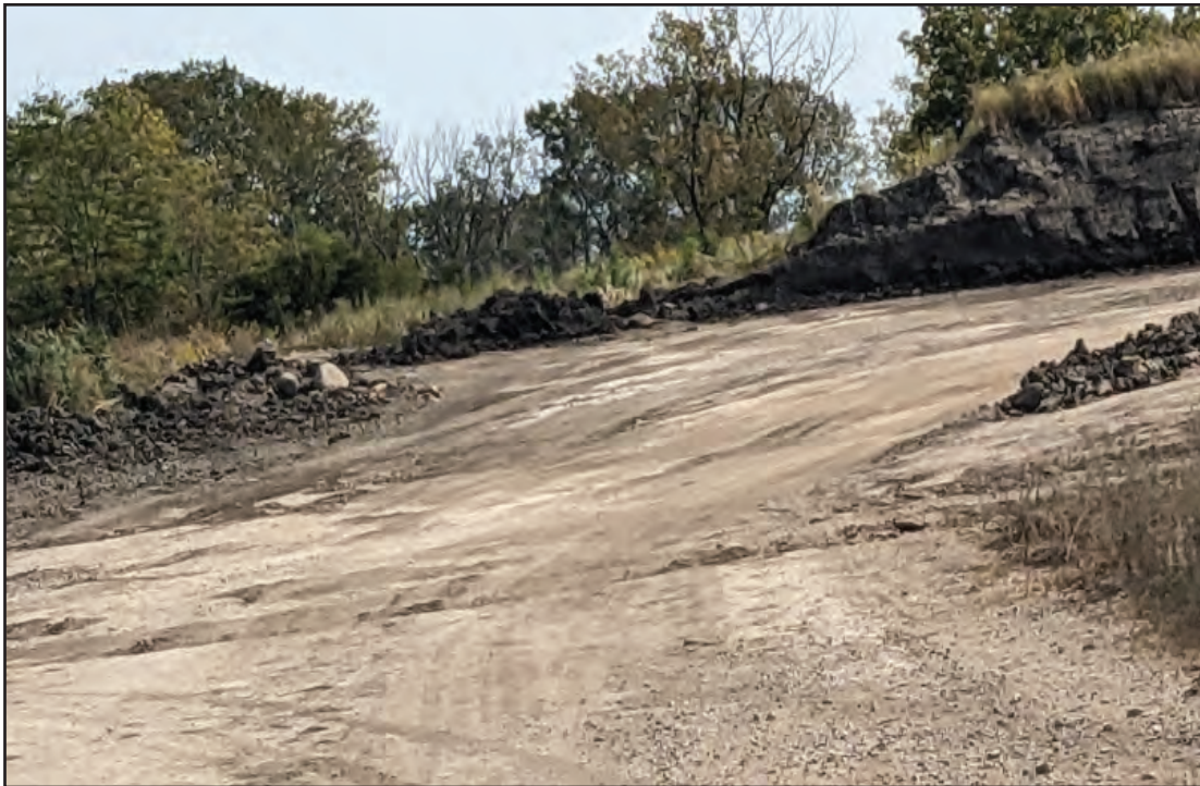
Site roads dry and stable
