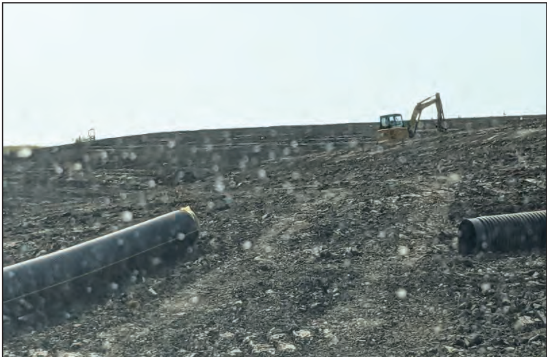
Stormwater controls being constructed into the cap
