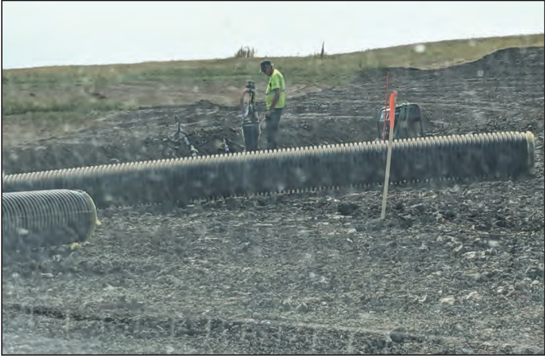
Stormwater controls being constructed into the cap
