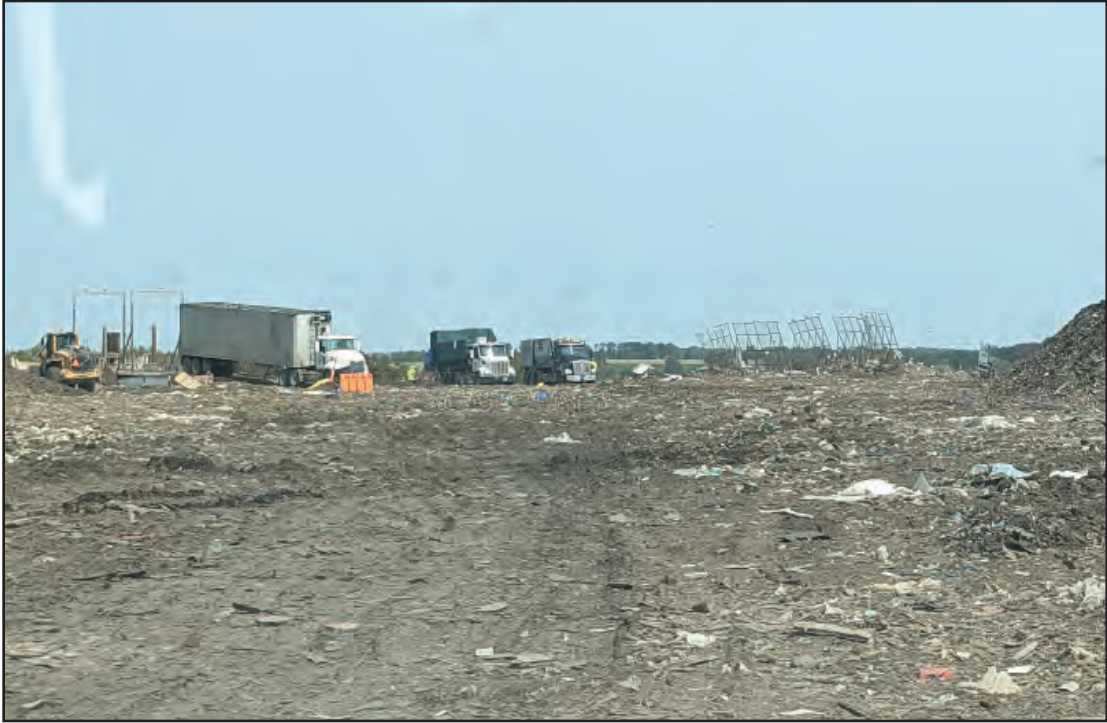
Travelway in active area improved with wood waste
