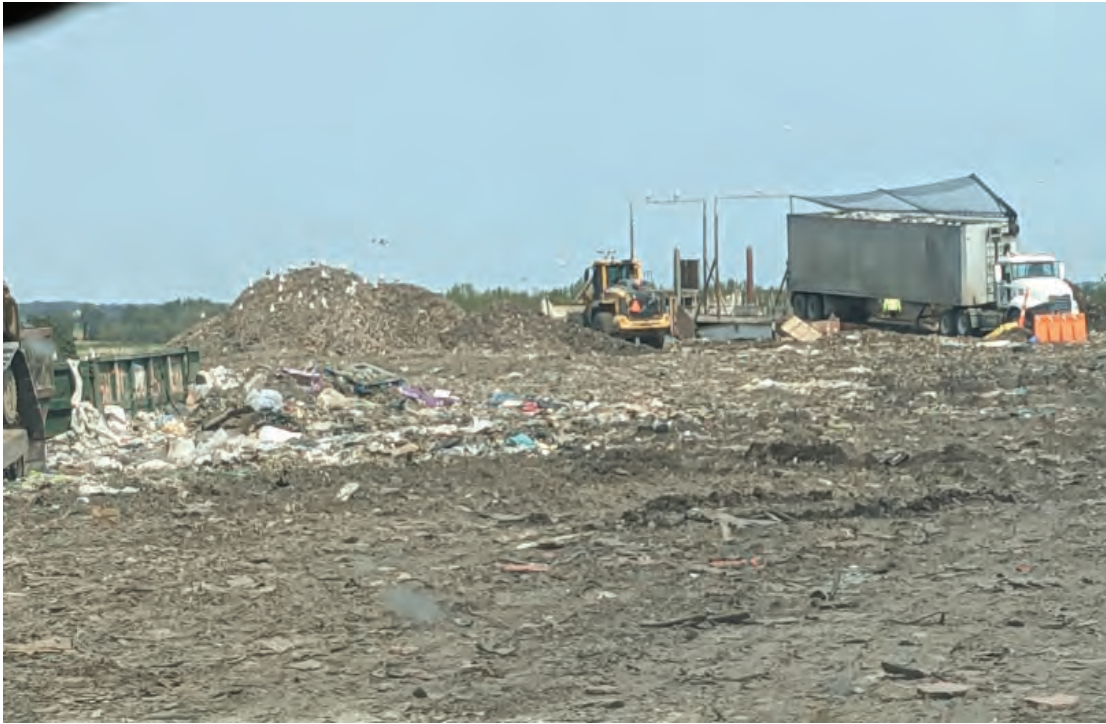
Clean out area and stockpile
